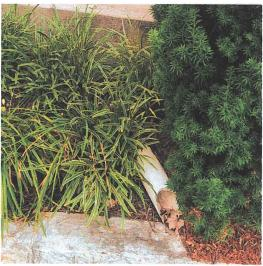
Both of these examples are immediately uphill from the Opera House. Leader at front of building connects to 4" pipe under sidewalk, daylights above curb.
