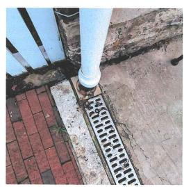
This is the typical configuration -- some with multiple leaders into a single slot. The opening at the curb is a concrete block with 2 slots (frequently clogged). Example at 112 West German (Bistro) shows leader displaced (water flows along building foundation).
